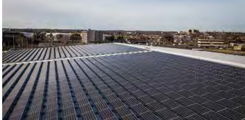
The solar panels are divided across two sections on the roof of CDI's 140,000 square foot facility in Stratford. Photo by Joe Palisi.
